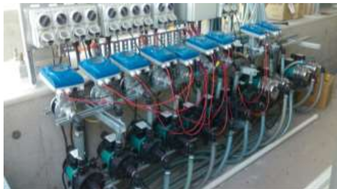
KMS502-25F 25mm flowmeters install
