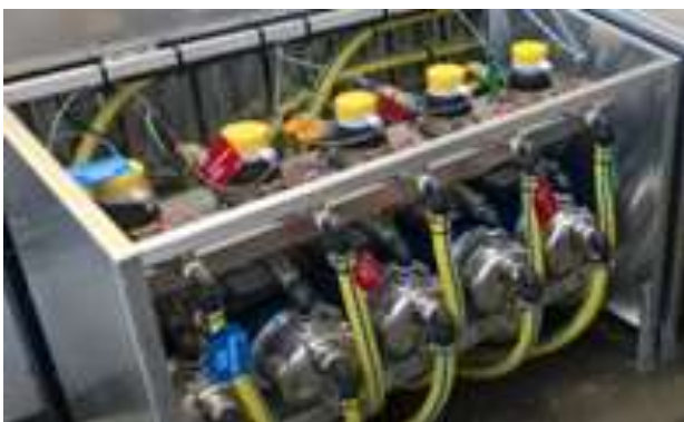
MES20 20mm flowmeters install
